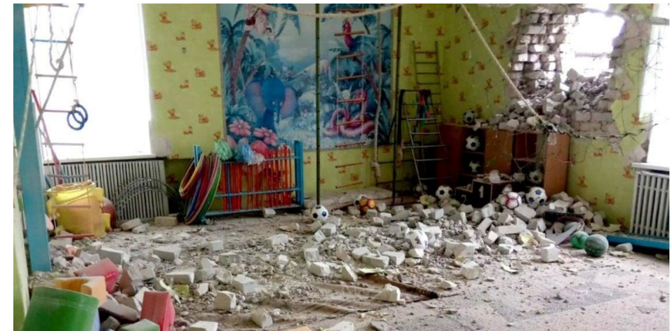
Destroyed kindergarten https://static.nv.ua/
